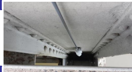
LIRIS Optical Strand on a bottom element
