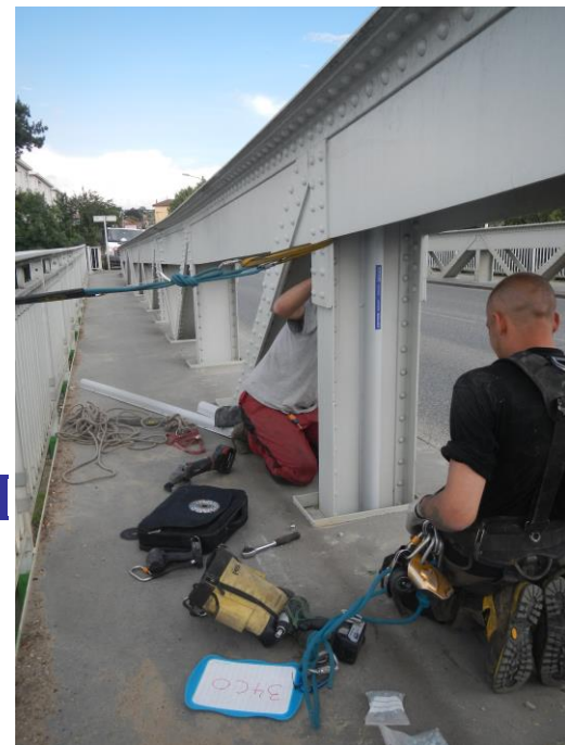
Installation of a LIRIS Optical Strand on a vertical unit
