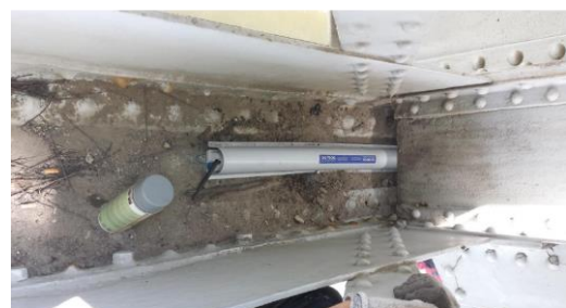
LIRIS Optical Strand on a bottom element with protection cover
